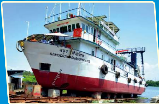
▲ Annual Survey and dry dock repairs of RV Samudra Shaudhi Kama at SBSL Slipway
